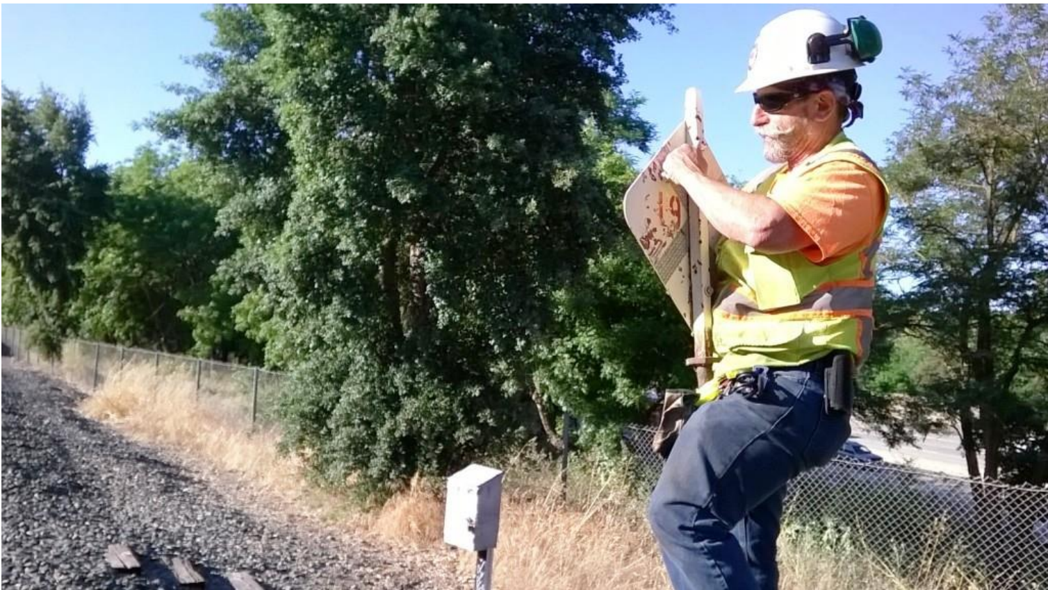
Joe removing an old switch target from the stand at Switch 19
