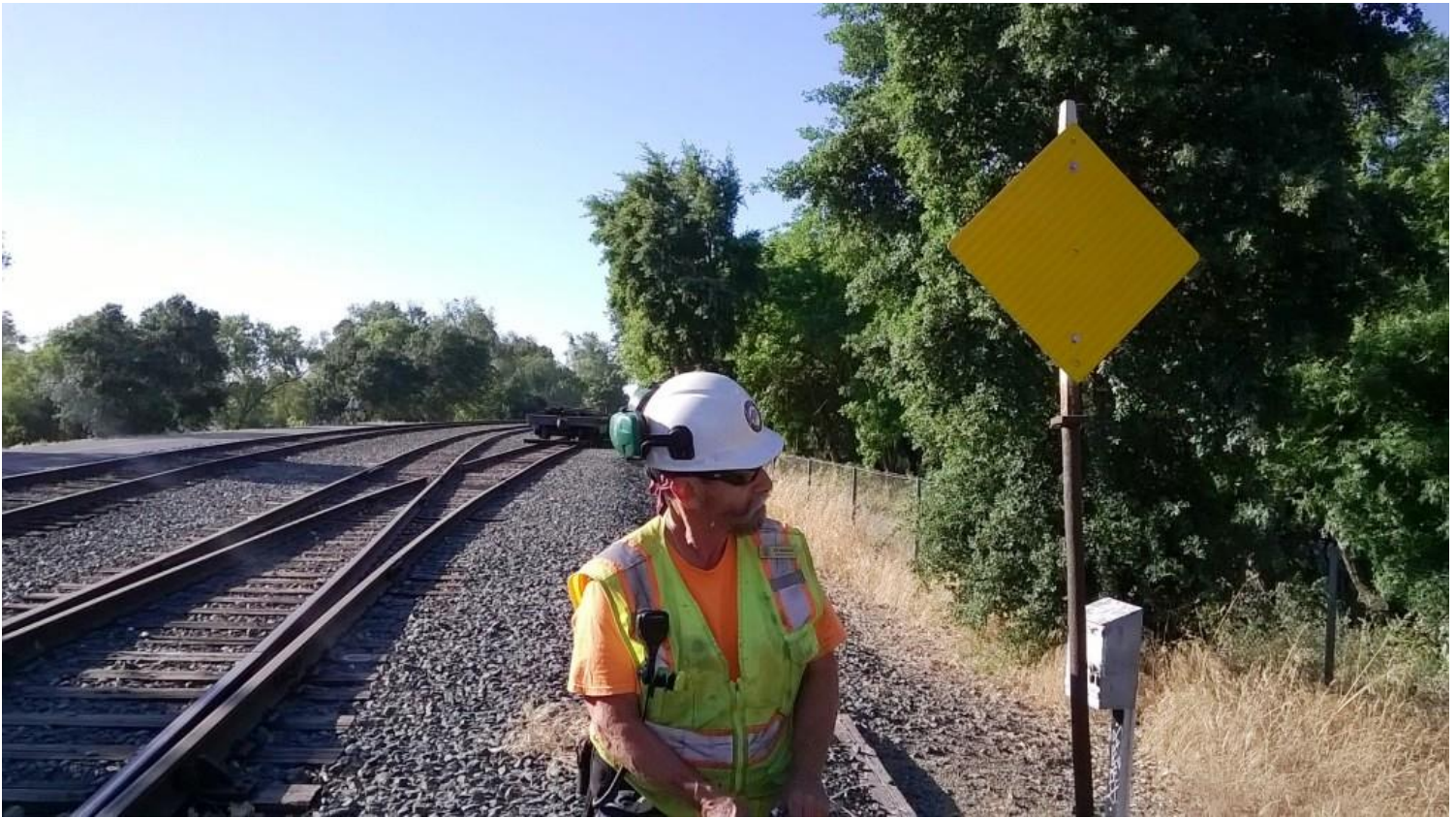
Joe admires the new fully reflective, graffiti-resistant switch target at Switch 19
