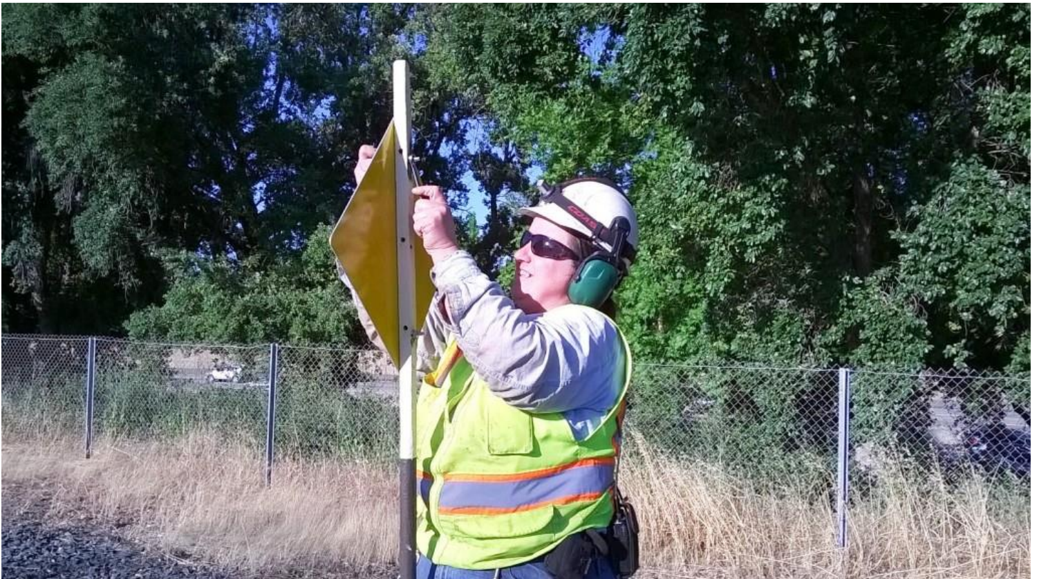
Heather replaces the switch target at Switch 18
